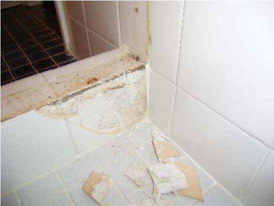
1. Remove existing wall tiles
