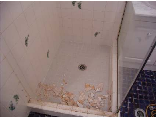
2. Removal of wall tiles and remove floor tiles
