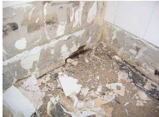
4. Repair or replace broken wall sheeting if required
